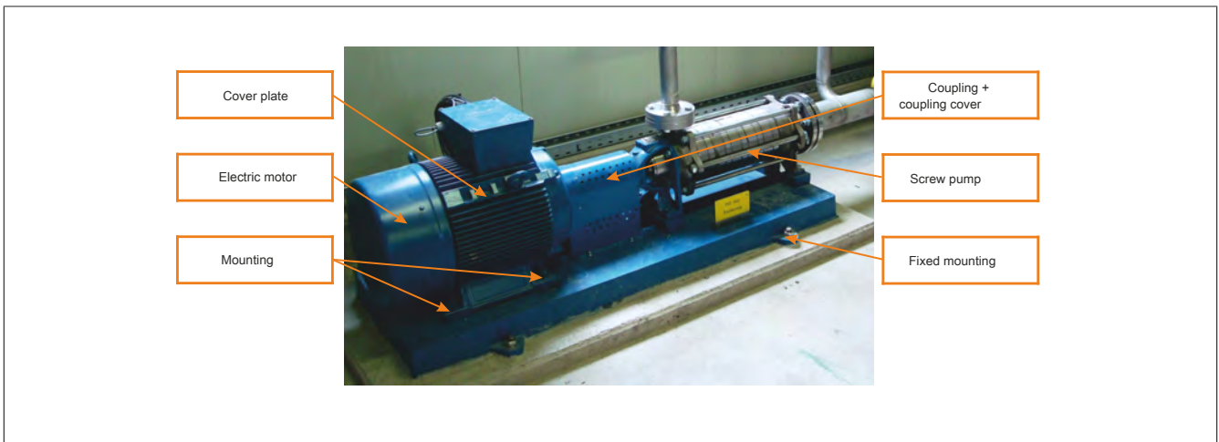
Figure 471: Structure of a pump drive
